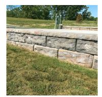
Created from architectural-grade, wetcast concrete, Kingstone blocks provide an aesthetically pleasing and structurally sound solution.
